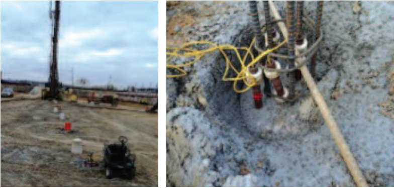
Installation of auger cast piles.
