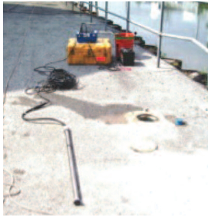
NDT Corporation uses a down hole magnetic gradiometer to determine the depth to the end of the pile.
