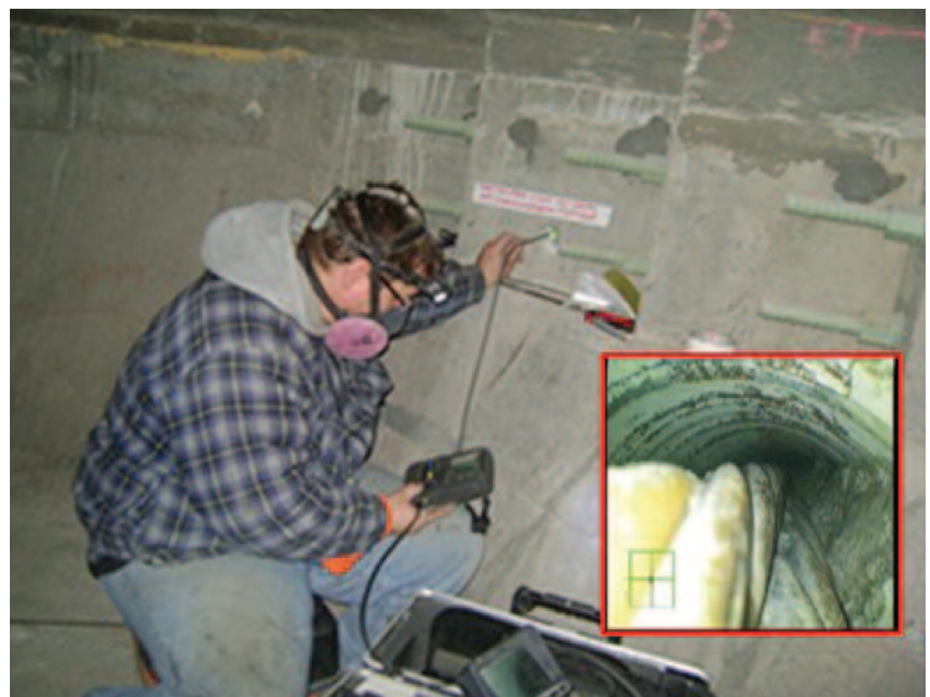
Documentation of a PT duct void via a borescope inspection.
