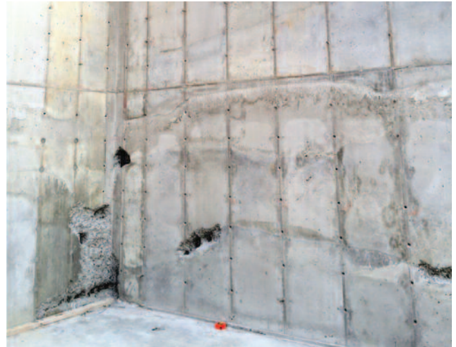
Pulse velocity measurements determined the extent of the weak areas in the recently poured concrete.
